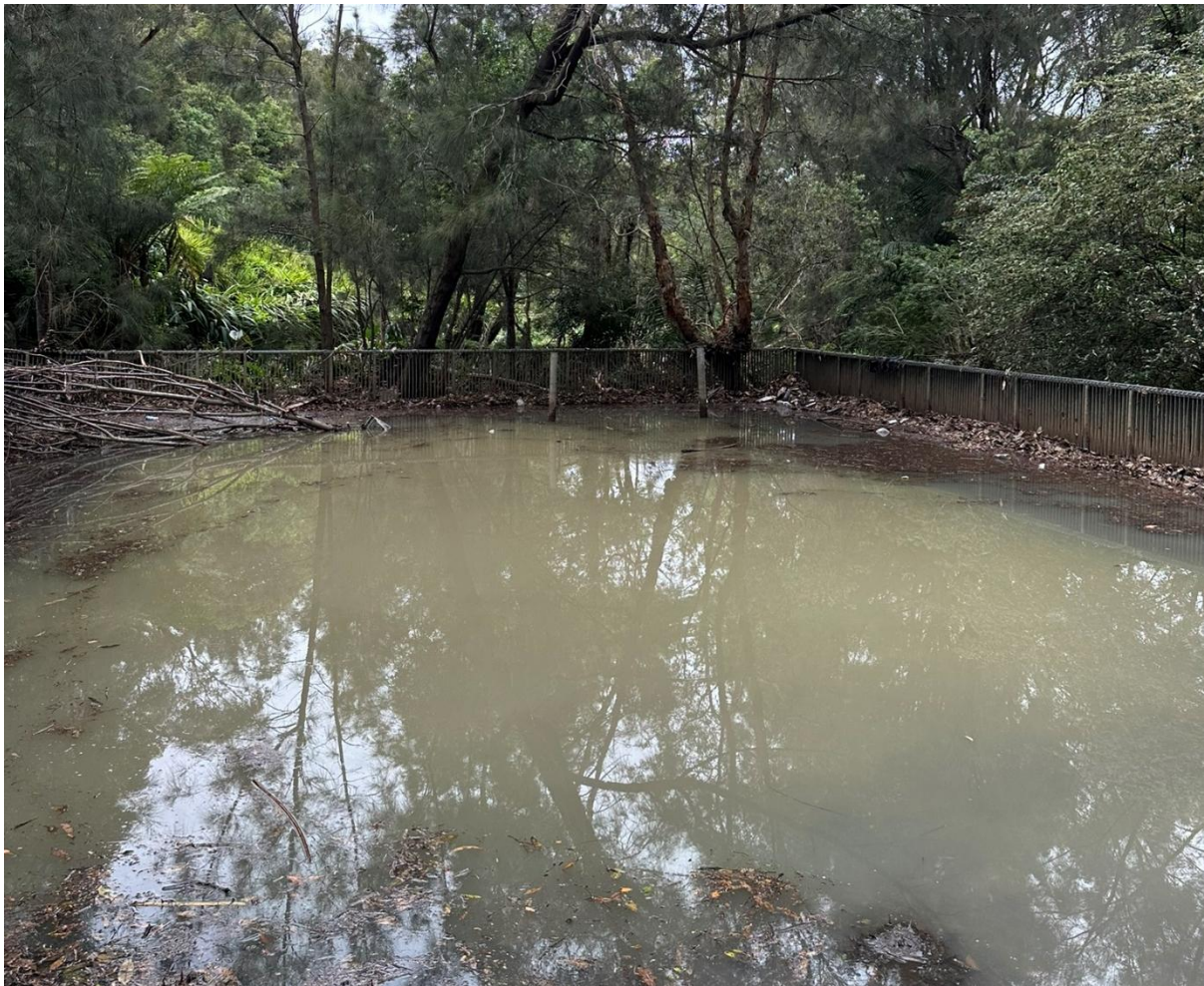
Figure 14. The current state of the existing trash rack (photo taken 16/10/2024)
