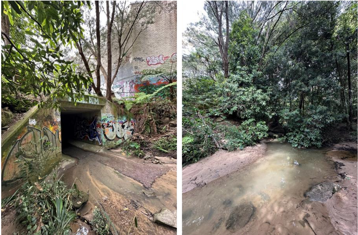
Figure 5. The interface between the piped and daylighted sections of Brookvale Creek at the eastern border of Allenby Reserve (ID 1 Figure 4 ). From left to right: a) Culvert: estimated dimensions 3.05m (W) x 3.0m (H). b) Well-vegetated area facing toward the upper reaches of Brookvale Creek from the same location as the culvert.
