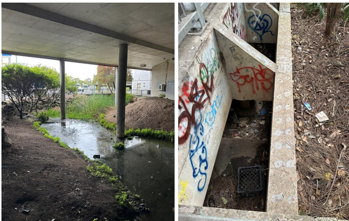
Figure 7. Entry of Brookvale Creek into the existing constructed waterway of the Warringah Mall stormwater system (ID 3 Figure 4). From left to right: a) Brookvale Creek flows into the existing culvert looking towards the entrance to Palm Tree Carpark. b) Overflow weir crest; entry to new culvert occurs in cases of overflow from the existing culvert adjacent to the Woolworths dock.
