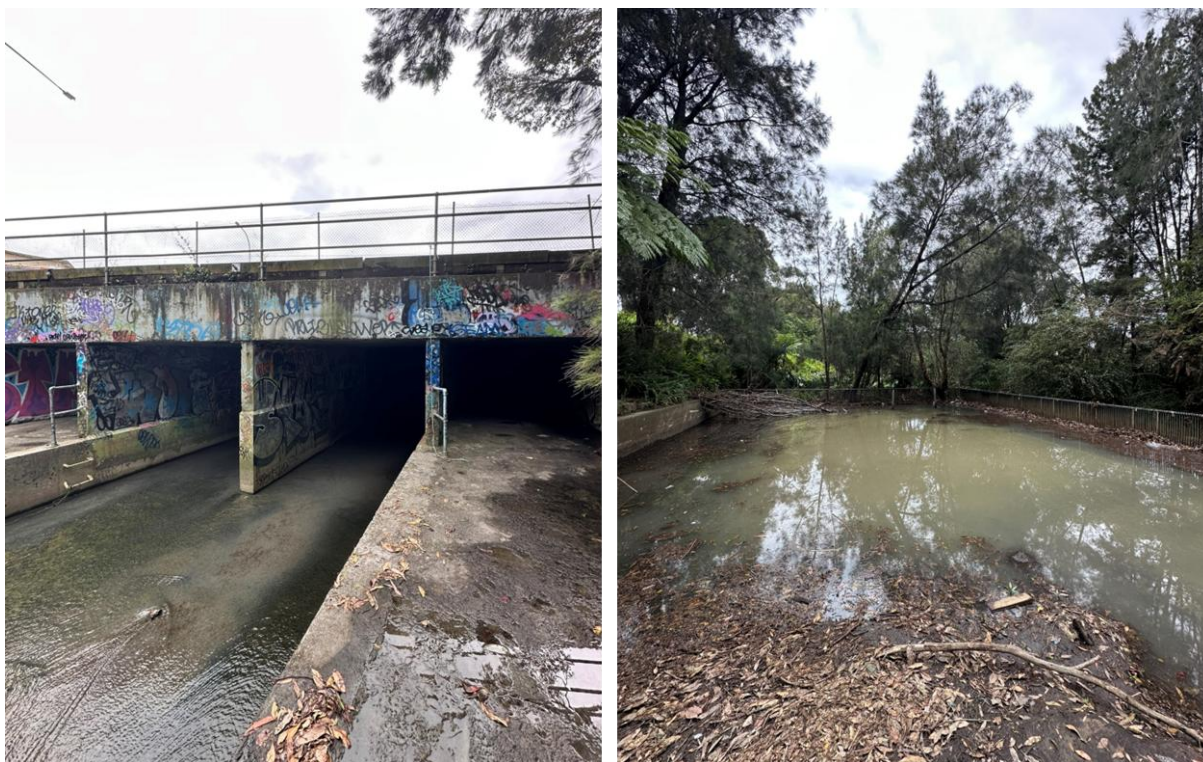
Figure 8. The interface between the piped and daylighted sections of Brookvale Creek along Condamine Street (ID 4 Figure 4). From left to right: a) Opening of culverts into Brookvale Creek. b) Trash rack downstream from culverts in Warringah Golf Club.
